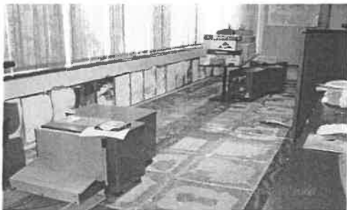
2. Typical office drywall removal.
