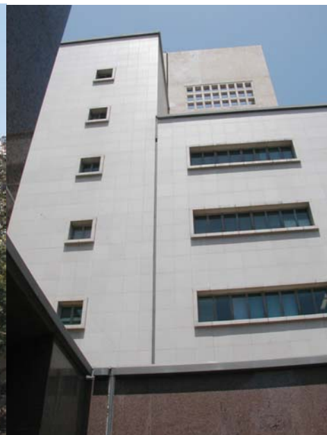
Seismic joint viewed from the south courtyard
