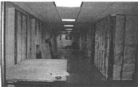
1. South hallway drywall removed.
