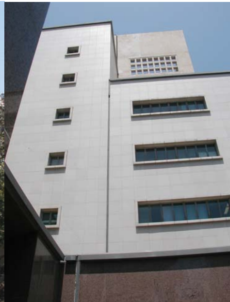
Seismic joint viewed from the south courtyard
