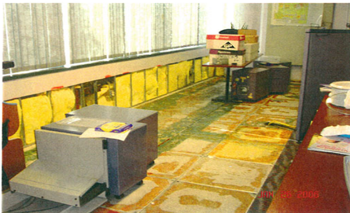
2. Typical office drywall removal.
