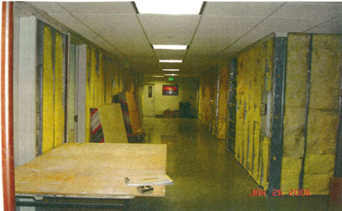
1. South hallway drywall removed.
