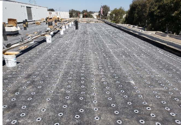
North County Regional Center - San Diego - Roof
