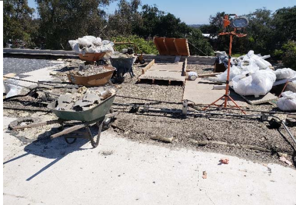
North County Regional Center - San Diego - Roof
