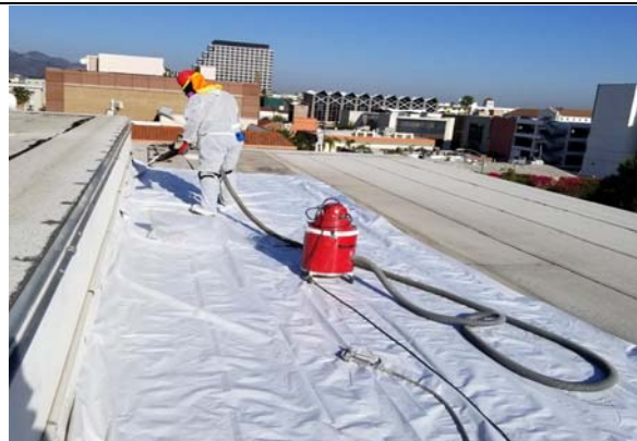
Glendale Courthouse - Glendale - Roof
