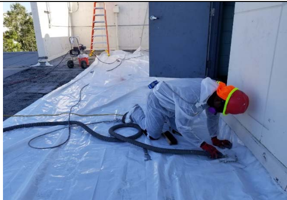
Glendale Courthouse - Glendale - Roof
