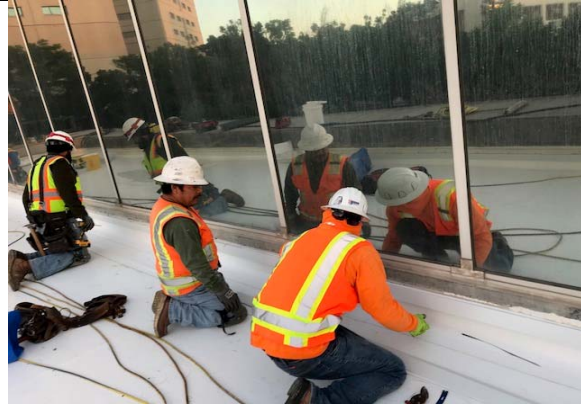
Hall of Justice East - San Jose - Roof
