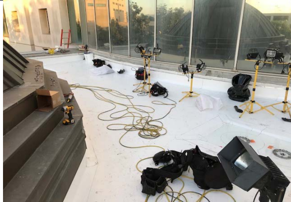
Hall of Justice East - San Jose - Roof
