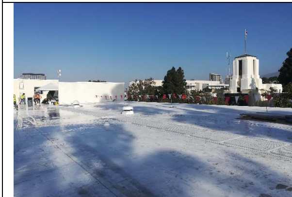
Glendale Courthouse - Glendale - Roof
