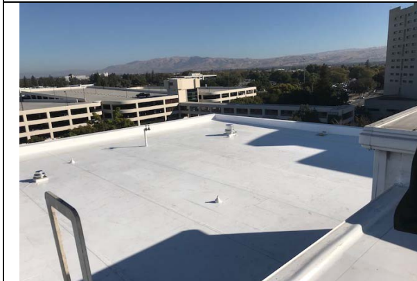
Hall of Justice West – San Jose - Roof
