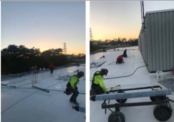
North County Regional Center - San Diego - Roof
