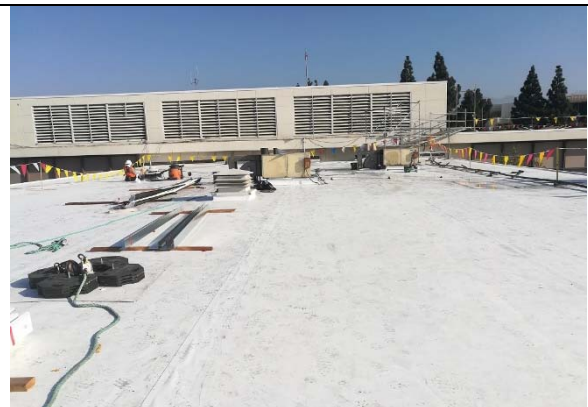
Glendale Courthouse - Glendale - Roof
