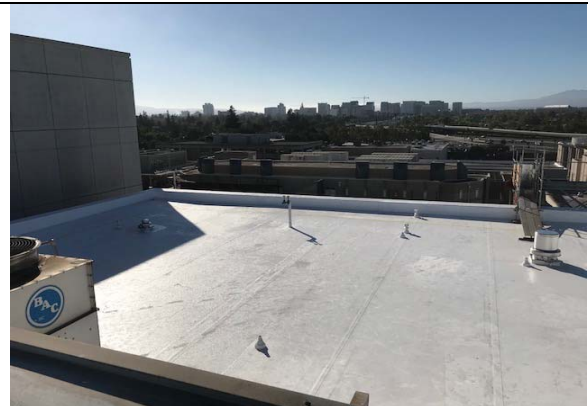
Hall of Justice West – San Jose - Roof
