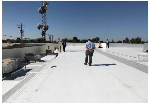
Shafter/Wasco Courts- Kern - Roof
