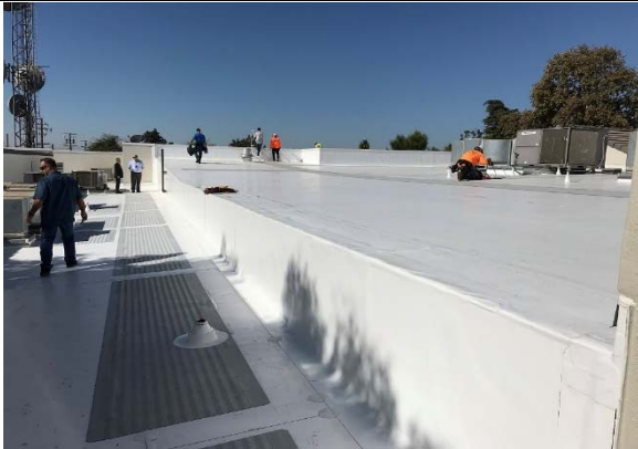
Shafter/Wasco Courts - Kern - Roof
