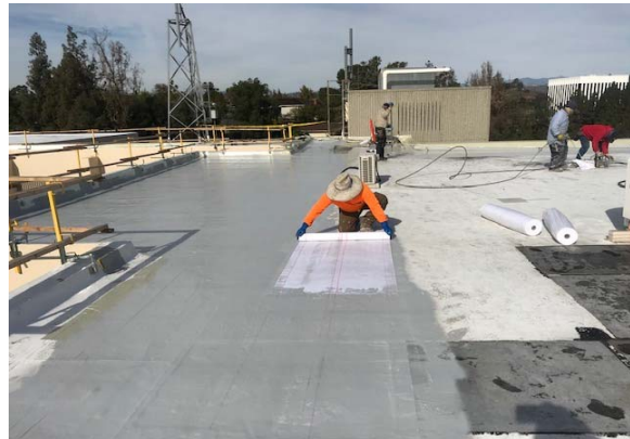
North Justice Center - Fullerton - Roof
