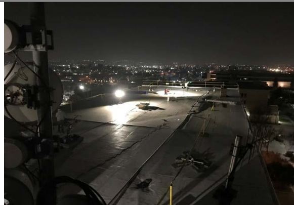
Bakersfield Superior Court - Kern - Roof
