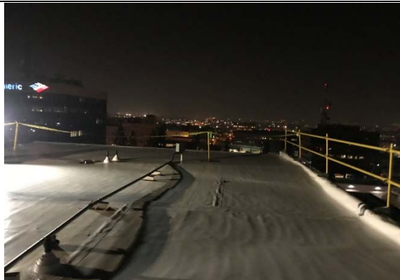
Bakersfield Superior Court - Kern - Roof
