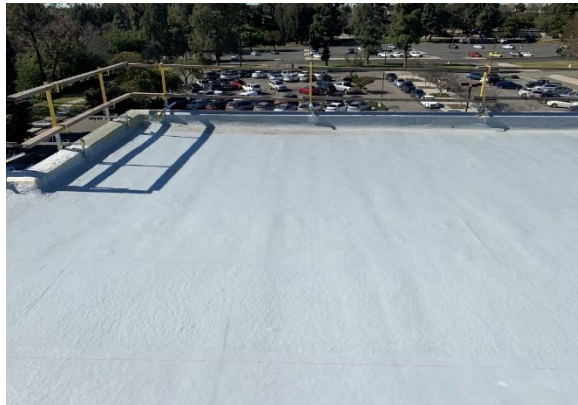
North Justice Center - Fullerton - Roof
