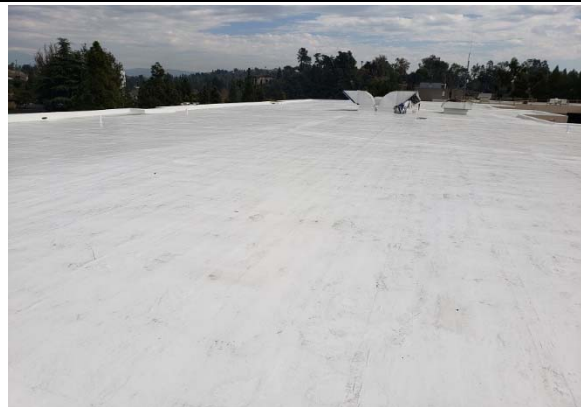
North Justice Center - Fullerton - Roof
