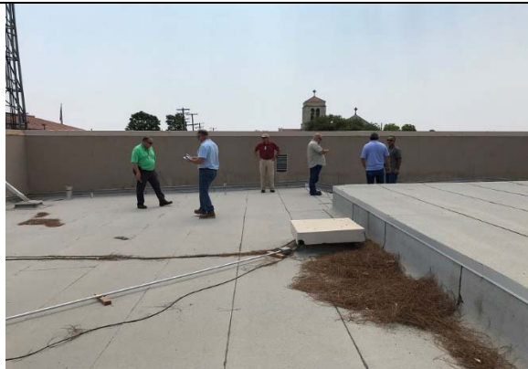
Delano Courthouse – Kern - Roof
