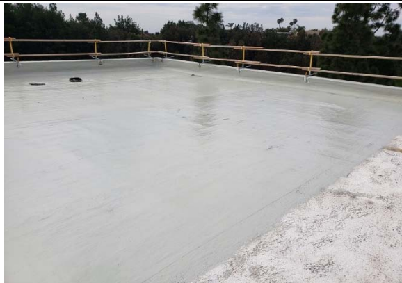
North Justice Center - Fullerton - Roof
