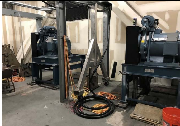
Edelman Children's Court - LA - Elevator
