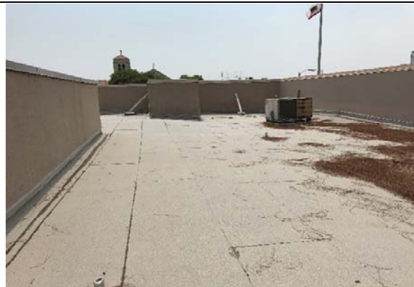
Delano Courthouse – Kern - Roof
