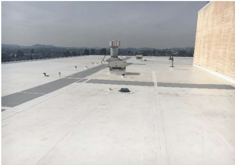
Below: Replaced roof with Class-A fire rated, 80 mil, PVC single-ply membrane
