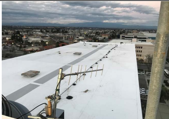
Bakersfield Superior Court - Kern - Roof
