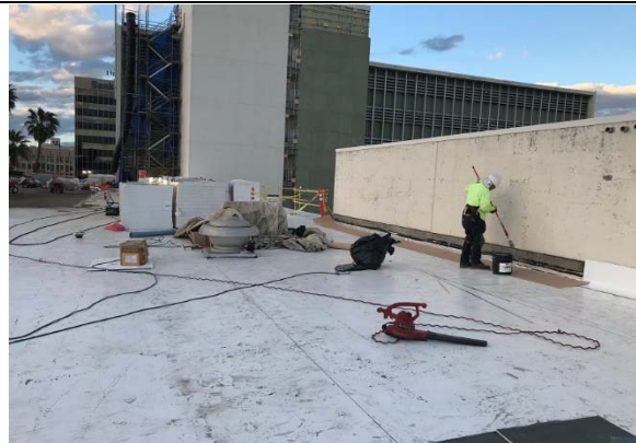
Bakersfield Superior Court - Kern - Roof
