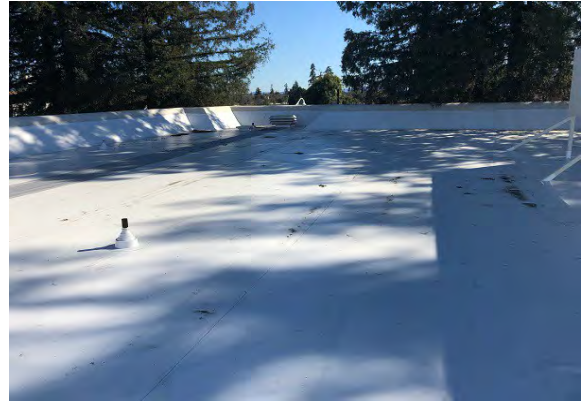
Santa Clara Courthouse - Santa Clara - Roof
