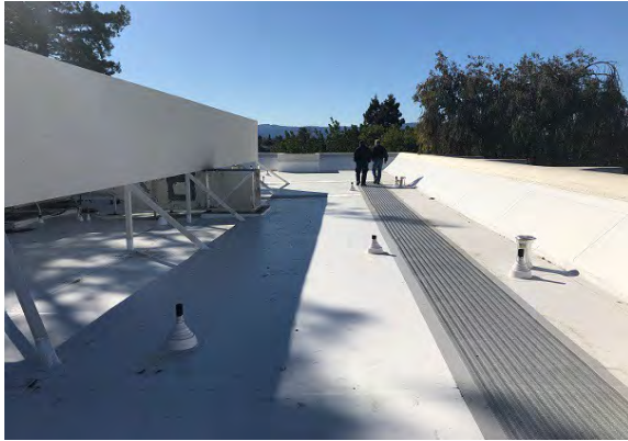
Santa Clara Courthouse - Santa Clara - Roof
