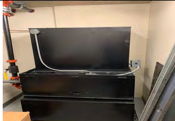
Burbank Courthouse - LA - Elevator
