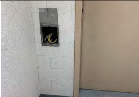
Burbank Courthouse - LA - Elevator
