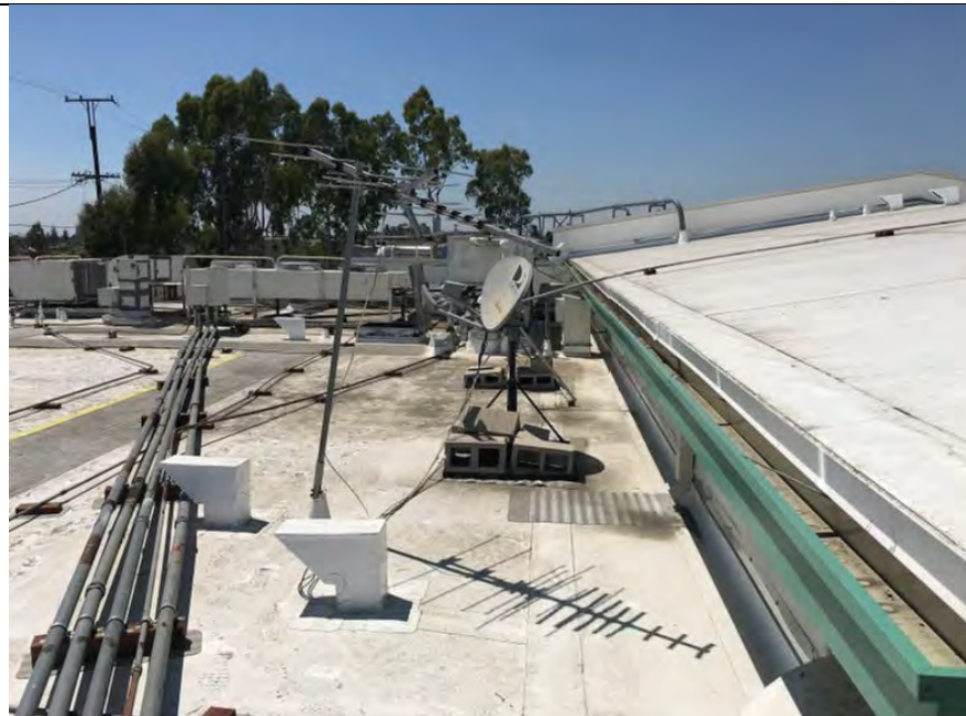
Newly replaced SBS roofing system with restored roof drains
