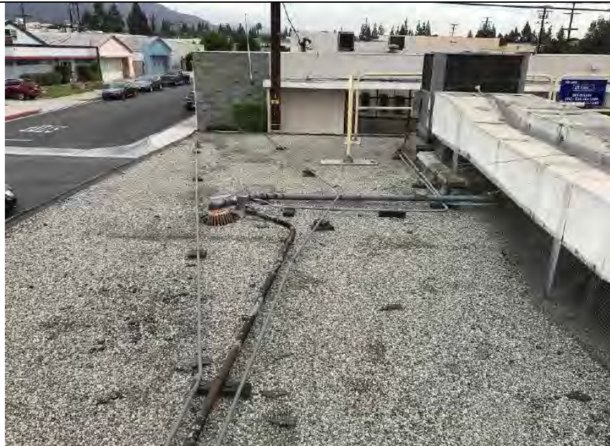
Old and failing built-up roof
