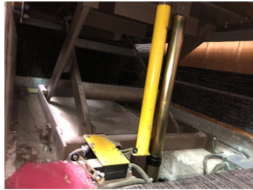
Downey Courthouse – Wheelchair lift refurbished hydraulic shaft
