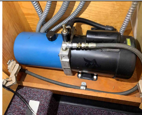
Bellflower Courthouse – Wheelchair lift refurbished motor
