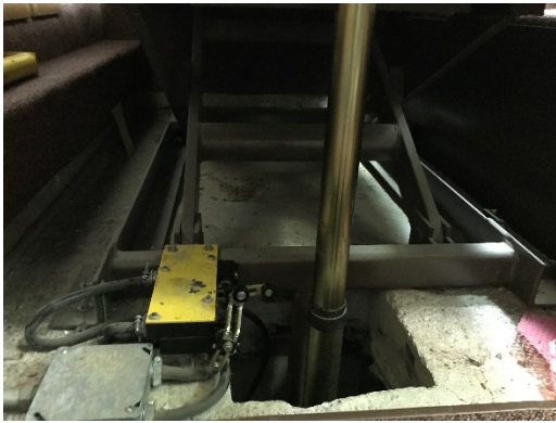
Downey Courthouse – Wheelchair lift old hydraulic shaft
