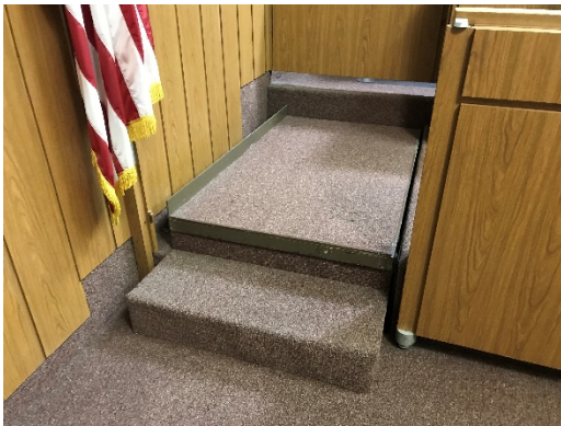
Downey Courthouse – Old Wheelchair Lift
