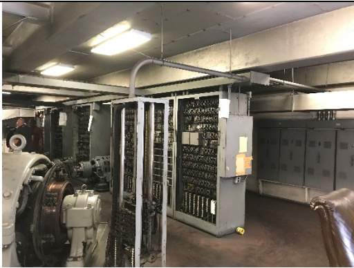
Stanley Mosk Courthouse Elevator Machine Room - Before
