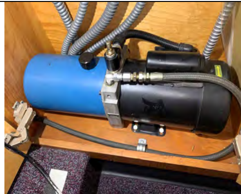
Bellflower Courthouse – Wheelchair lift refurbished motor
