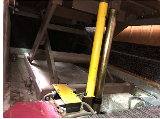
Downey Courthouse – Wheelchair lift refurbished hydraulic shaft
