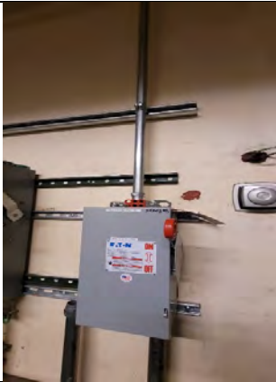
El Monte Courthouse – Elevator 5 New
