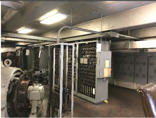
Stanley Mosk Courthouse Elevator Machine Room - Before
