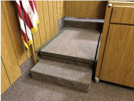
Downey Courthouse – Old Wheelchair Lift
