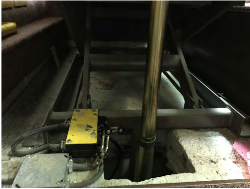
Downey Courthouse – Wheelchair lift old hydraulic shaft
