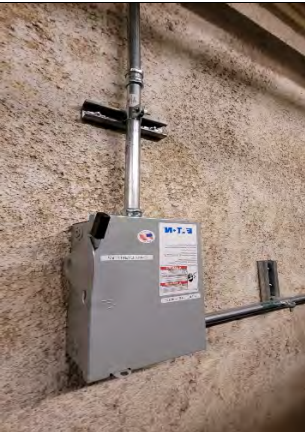
El Monte Courthouse – Elevator #2
