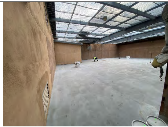
East County Regional Center – Roof
