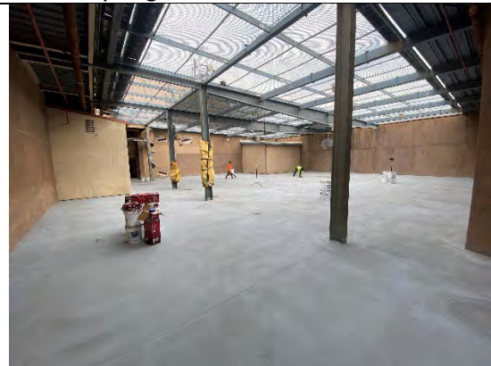
East County Regional Center – Roof
