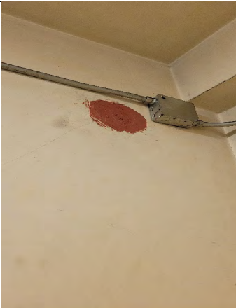
El Monte Courthouse – Elevator
