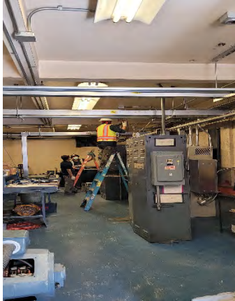
El Monte Courthouse – Elevator
