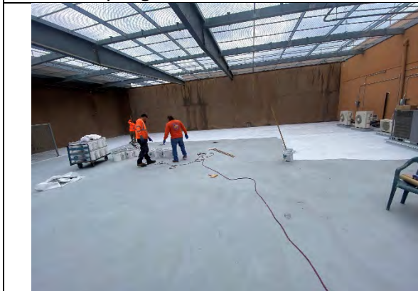
East County Regional Center – Roof
