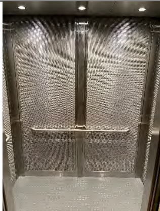
Walnut Creek Courthouse – New Elevator Cab
