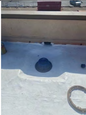
Kearny Mesa Court – New Drain Sump
