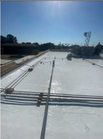
Kearny Mesa Court – New Roof
