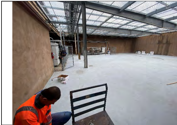
East County Regional Center – Roof
