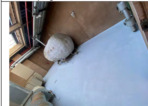
East County Regional Center – Roof
