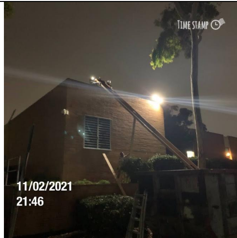
Torrance Annex Roof Replacement
