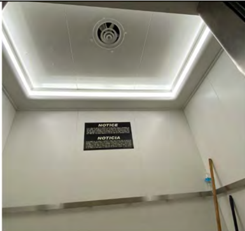
El Monte Courthouse Elevator Replacement
