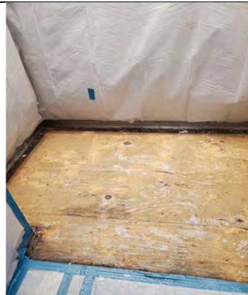
El Monte Courthouse Elevator Replacement
