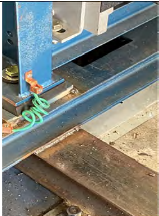
El Monte Courthouse Elevator Replacement
