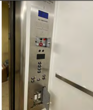
El Monte Courthouse Elevator Replacement
