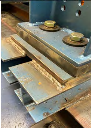
El Monte Courthouse Elevator Replacement
