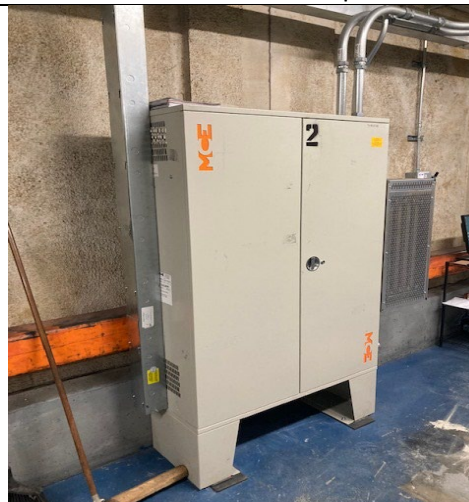
El Monte Courthouse Elevator Replacement
