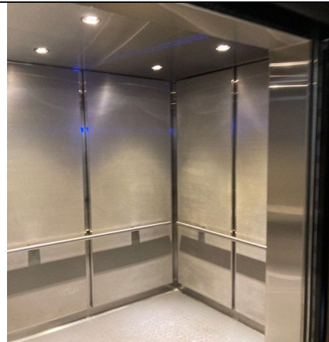
El Monte Courthouse Elevator Replacement
