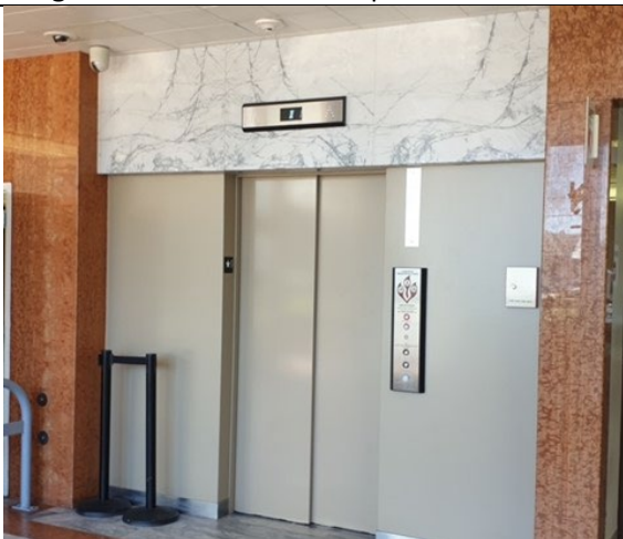
George D. Carroll Elevator Replacement (New)
