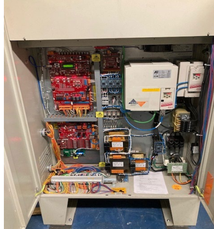
El Monte Courthouse Elevator Replacement
