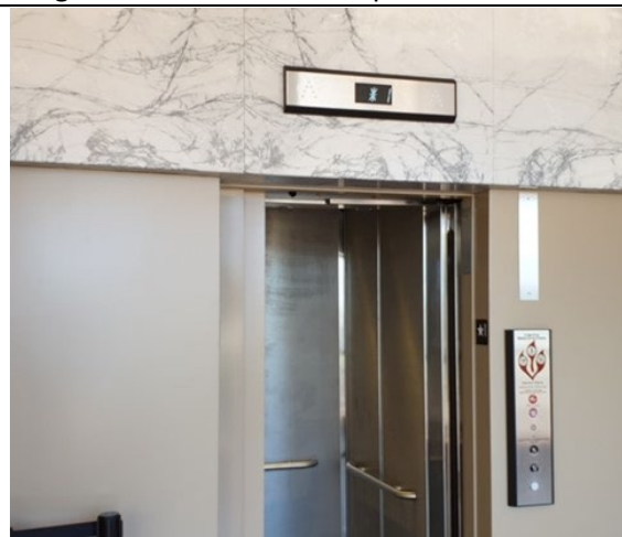
George D. Carroll Elevator Replacement (New)
