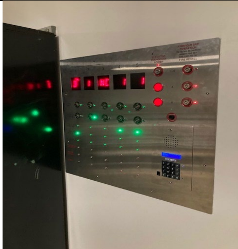
El Monte Courthouse Elevator Replacement
