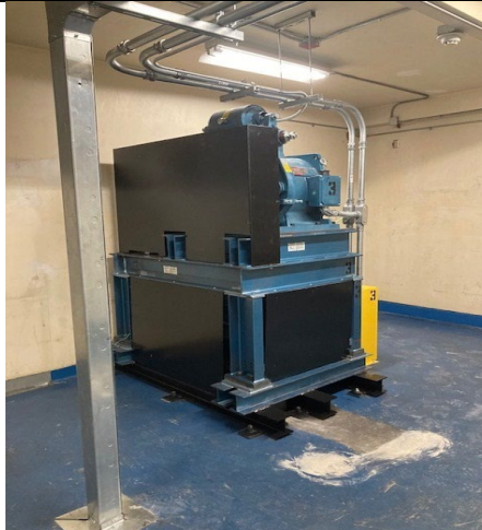
El Monte Courthouse Elevator Replacement
