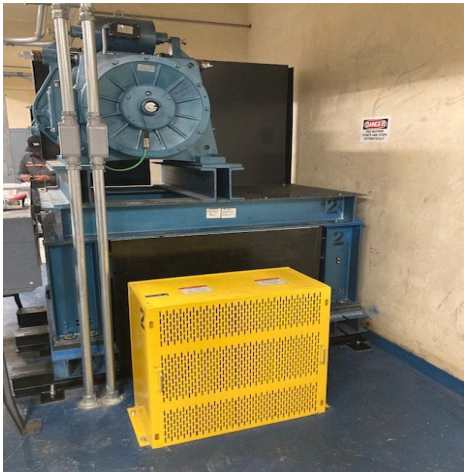
El Monte Courthouse Elevator Replacement
