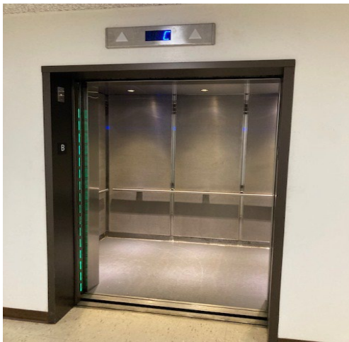
El Monte Courthouse Elevator Replacement
