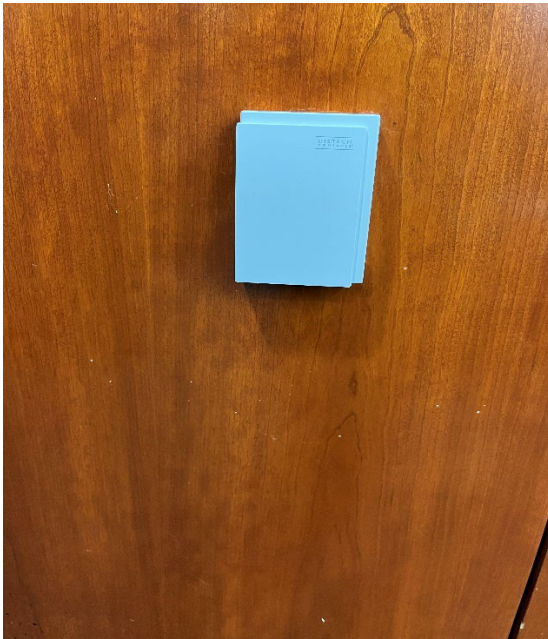
Criminal Court Building – BMS
