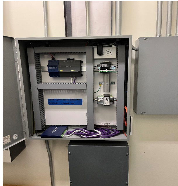
Criminal Court Building – BMS
