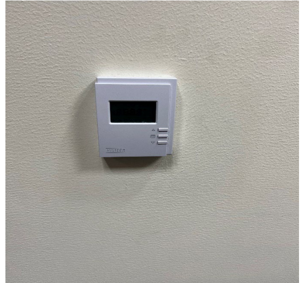
Criminal Court Building – BMS
