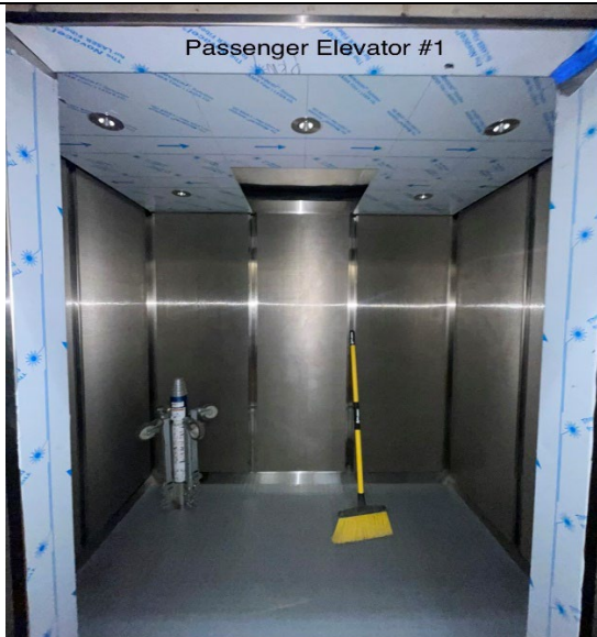
Fremont Hall of Justice - Elevator
