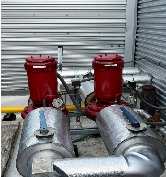
Criminal Court Building – BMS
