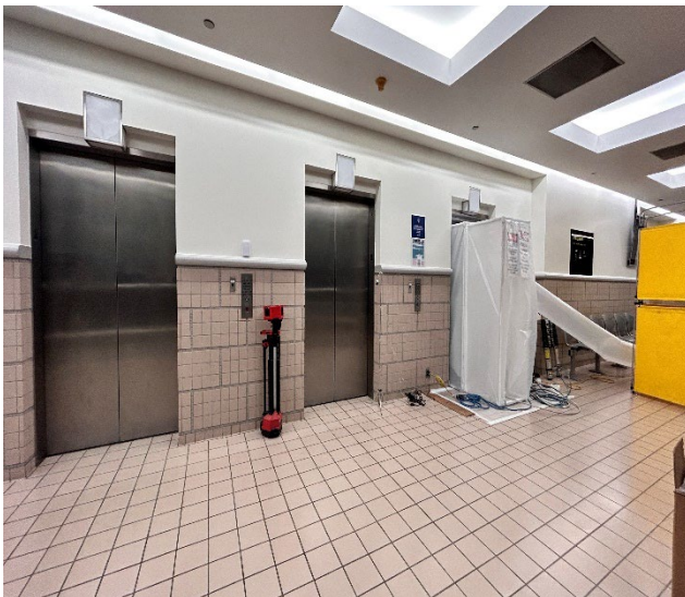
East Los Angeles Courthouse - Elevators
