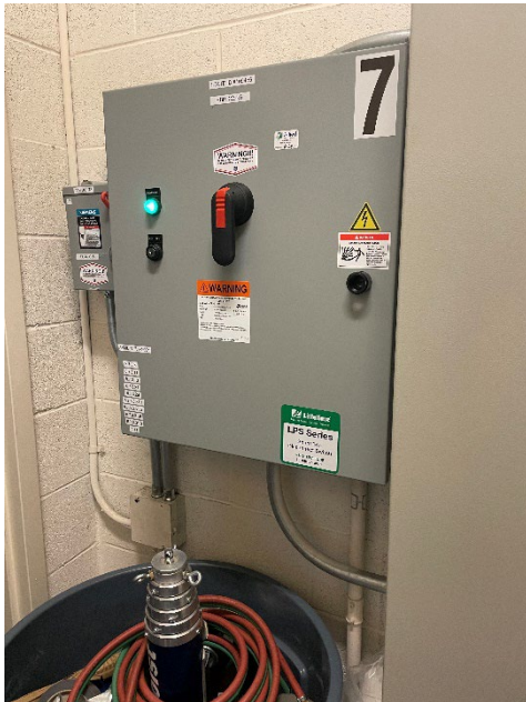
Civic Center Courthouse - Elevators
