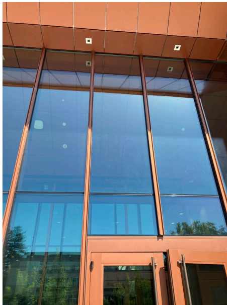
Newly replaced tempered glass windows at public entrance
