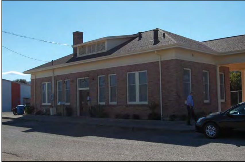
Depot Building. View to the southwest.
