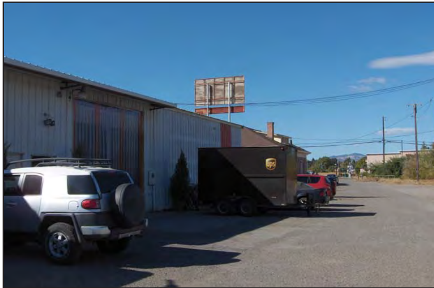
East side of Warehouse Building. View to the northwest.
