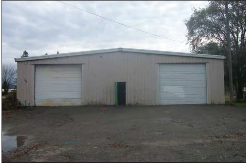
North side of Shop Building (307 E. Perkins). View to the south.
