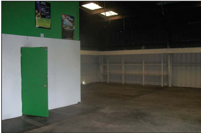
SW Interior of Shop Building. View to the southwest.
