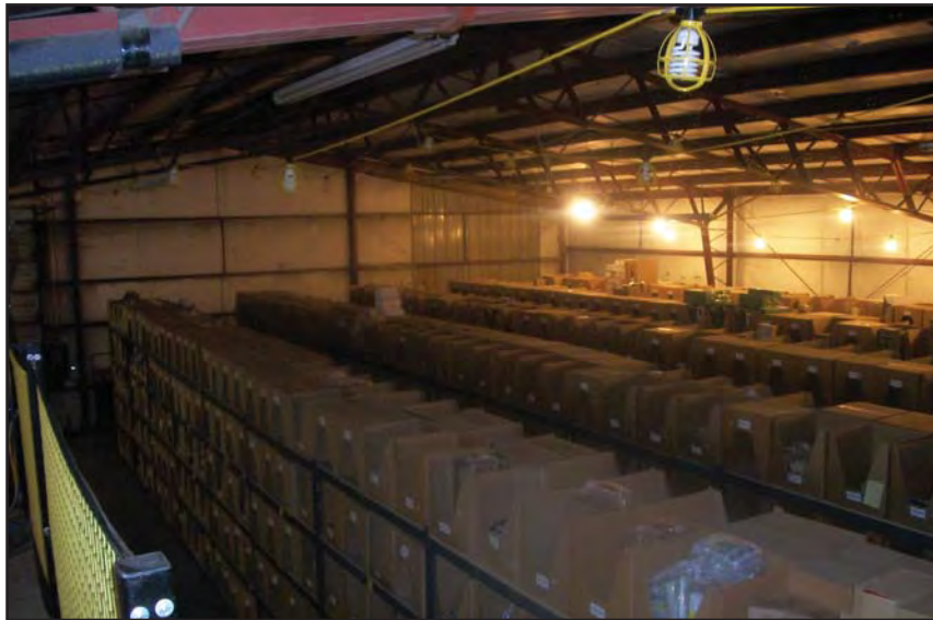
Southern Portion of Warehouse Building from loft. View to the south-west.
