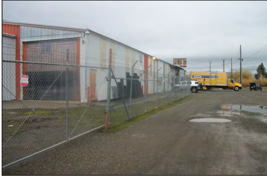
Exterior East Side of Shop Bldg. View to the north-northwest.
